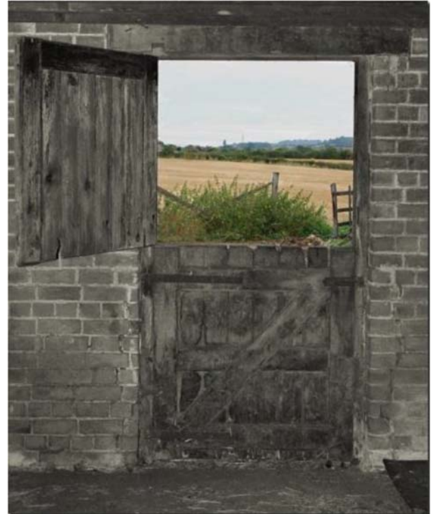
Figure 28. Pics & Photos (2014) View from inside the stable. Bottom Door Height 3' 6" (107cm) for standard donkeys and, ideally the door width should be 4' (122cm) [Photograph] Accessed from http://www.photographyblo.com
