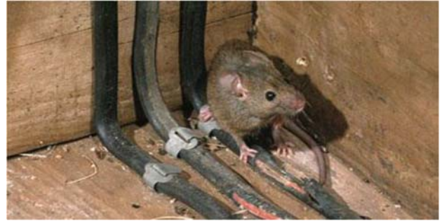
Figure 38. Security Pest Control. Ant-Termite-Bedbugs-Rodent Control MA (2014) House mice gnaw through electrical wiring causing fires and failure of stable appliances [Photograph] Accessed from http://www.securitypest.com/
