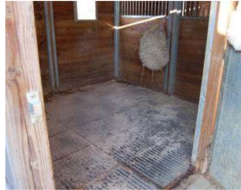
Figures 47 & 48. (Figure 47) Levade Systems & (Figure 48) Happy-Horse-Training.com (2011) (Figure 47) Rubber matting stable & (Figure 48) A rubber-floored box with little or no bedding may look to us bare an uncomfortable, but for a donkey it is more important for them to be properly protected from the unnaturally hard and cold surface of a concrete stable floor [Photographs] Accessed from (Figure 47) http://www.levadesystems.co.uk/ y (Figure 48) http://www.happy-horse-training.com
